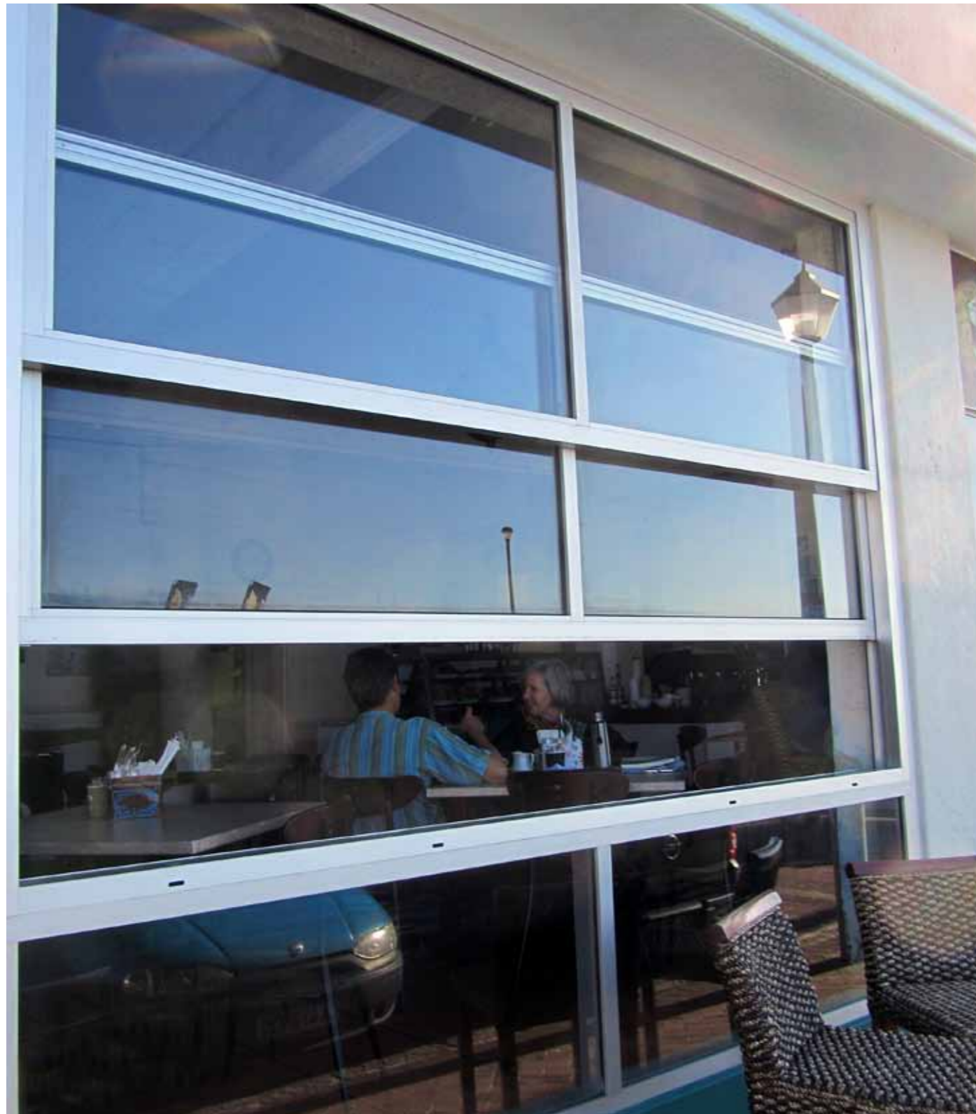
Gary's Surf Shop, Muizenberg Beachfront. Custom ISO100 Vertical Sliding Window with counterweights
