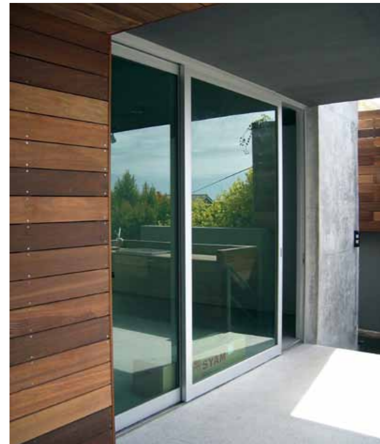
Residence, Fresnaye. Natural Anodized, Green tinted Glass
