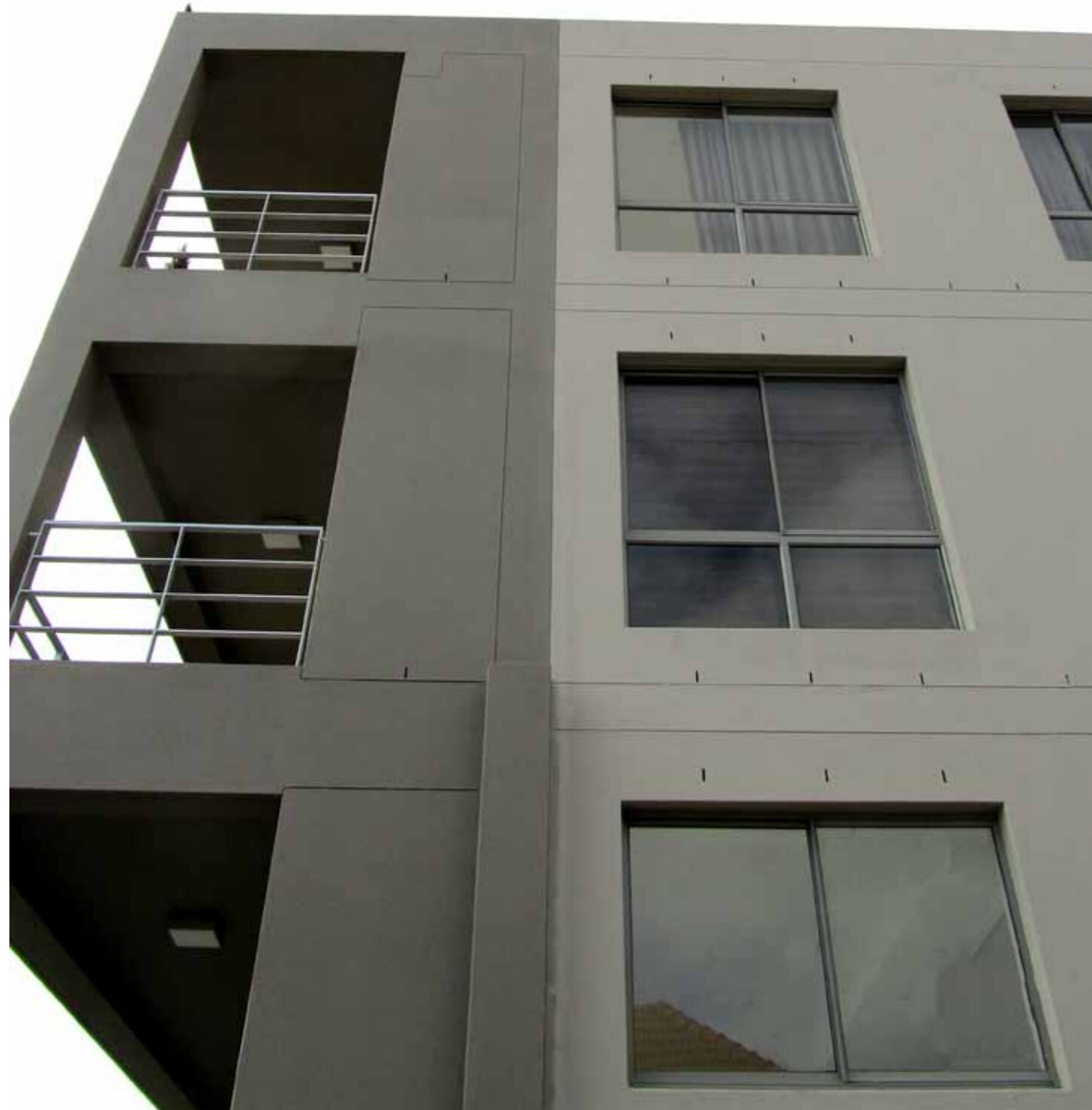
Chepstow Apartments, Chepstow Road. Sea Point. Powder Coating Stone Grey.
