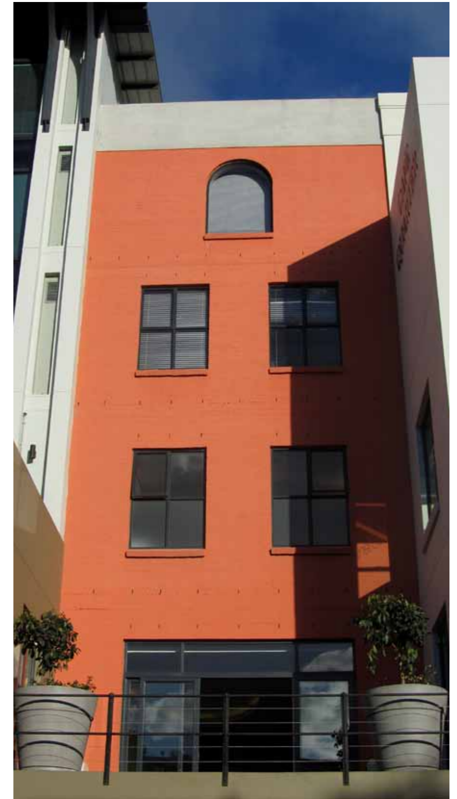
Cape Quarter Extension, Napier street, Cape Town
