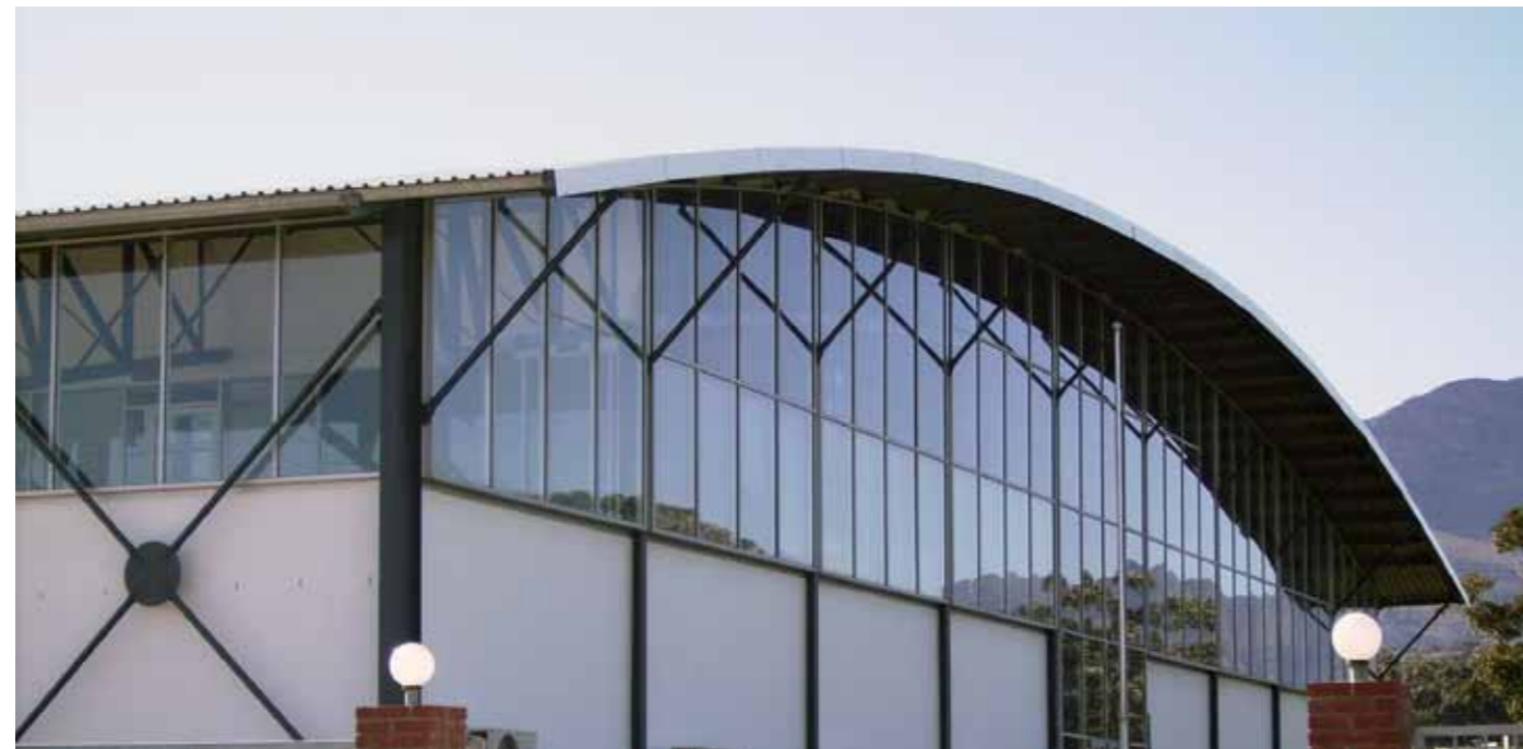
Olive Grove, Somerset West
