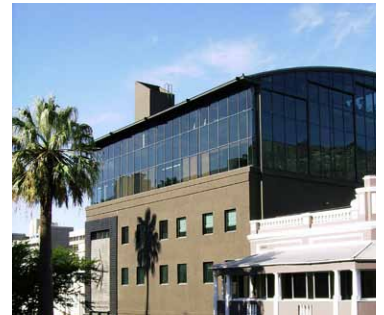
Renaissance Building, 199 Bree street, Cape Town. Solarvue green PVB laminated glass
